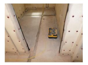
Figure (7) Membrane taped joints
