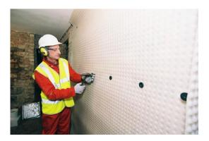
Figure (6) Membane plug fixings
