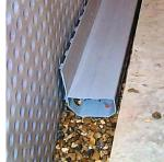
Figure (8) Typical perimeter drainage channel
