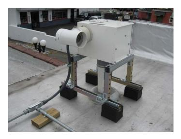
Figure 46, Example of AMG Force Installation
