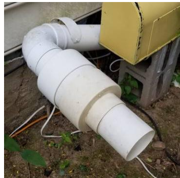
Figure 8: Corentium Pro installed in exhaust piping
