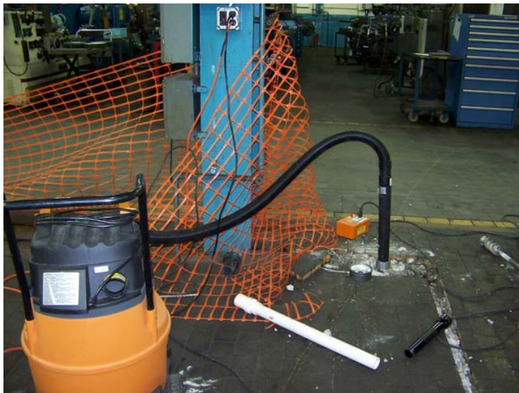
Figure 8 Sub-Slab Communication Test
